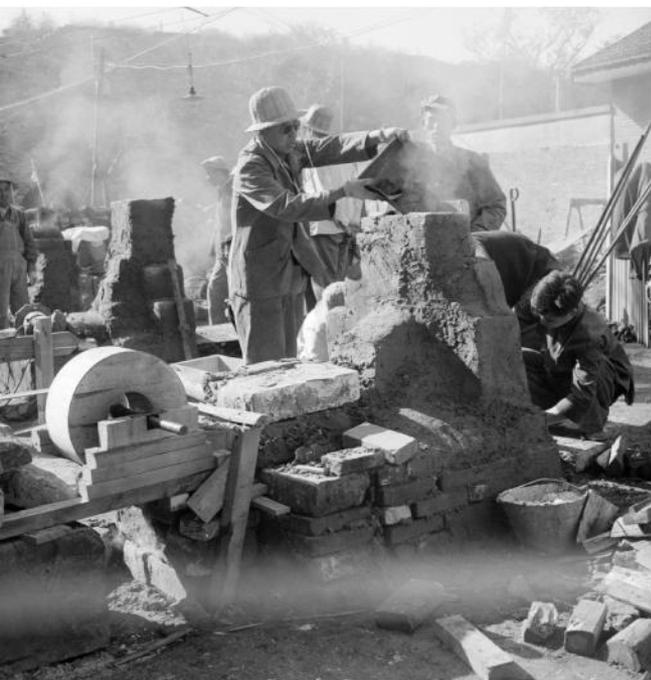
▲ Constructing a rudimentary smelting steel furnace, 1958
